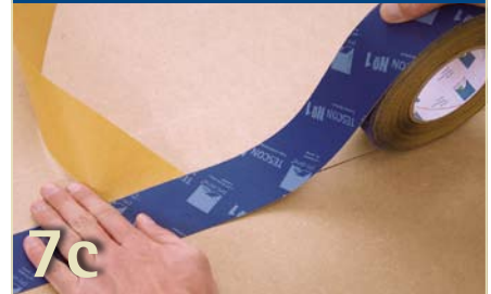
Sealing sarking boards
