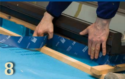
Sealing external junctions
