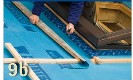
Details for underlay gutters
