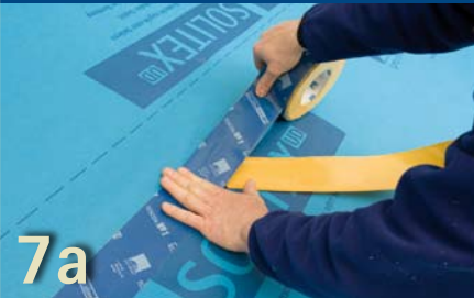
Taping roof underlay
