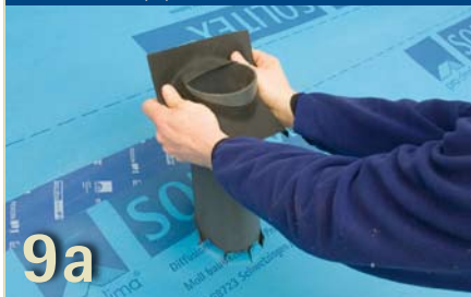
Details for pipes externally
