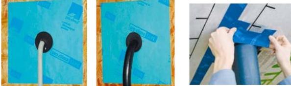
Grummets are made from non-ageing elastic EPDM and are available in a range of sizes from 6 up to 220mm. The grummets available are:
