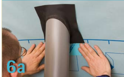
Details for sealing pipe ducts
