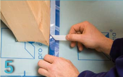
Details for taping corners
